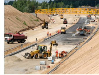
(a) Terrassements routiers
